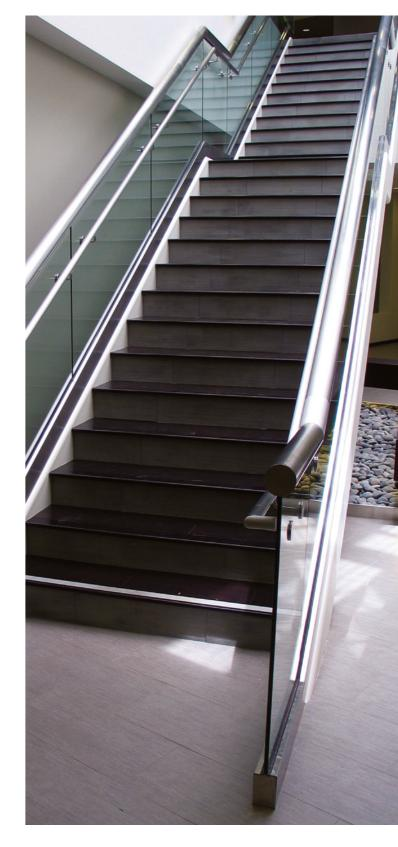
All the data included within this table is dependant on correct installation of the base shoe plus actual glass strengths. Based on 1100mm Balustrade Heights anchored 300mm on center to concrete or steel substrates.
