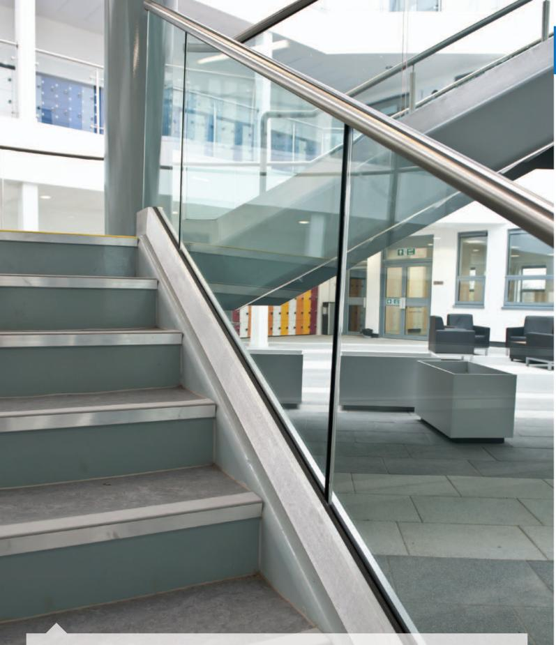
Aluminium Base Shoe for Toughened and Laminated Toughened Glass
